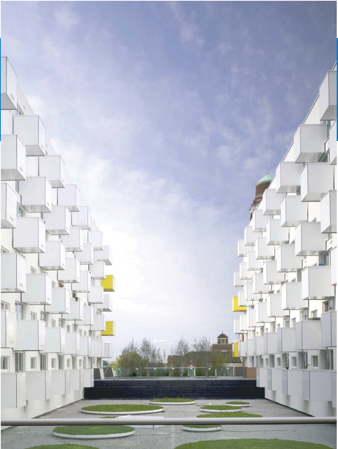
Project Management and Quantity Surveying. Barking Town Square, London – Joint venture between the private and public sectors transforming tired 1970s concrete framed library structure into mixed use amenity and constructing two new six storey blocks on top comprising 246 apartments with distinctive balconies and a shared rooftop garden.
